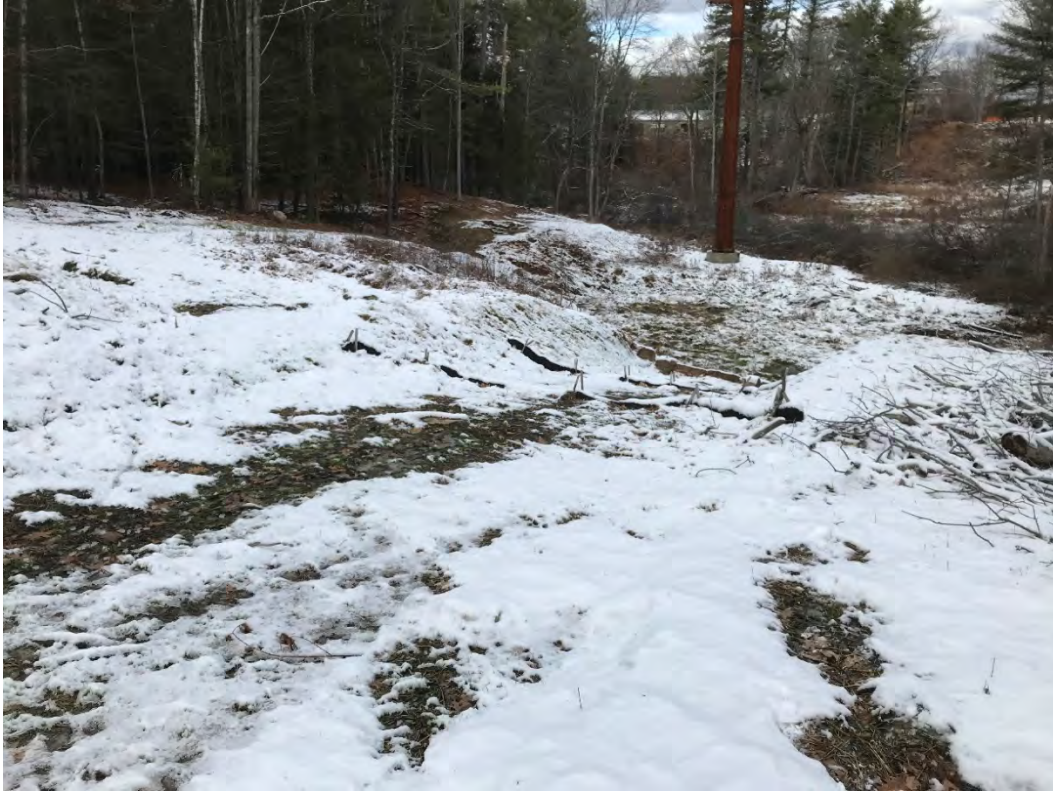
Fig 11: Lower portion of slope between Strs. 28 and 29. Viewing northwest. (12-07-20)
