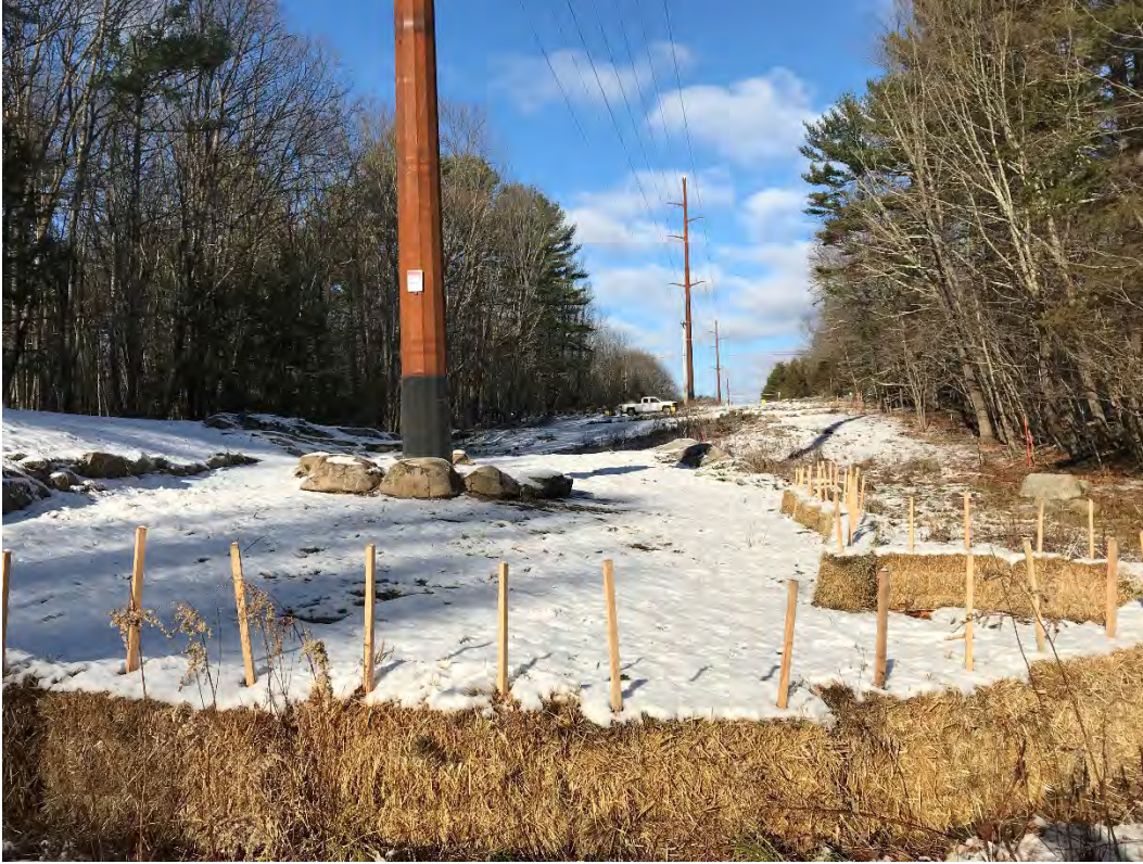
Fig 7: Str. 89 work area. Viewing northwest. (12-07-20)
